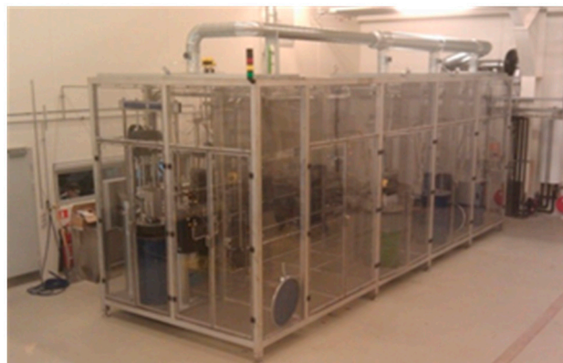
Figure 7. HTL plant. The completed HTL pilot plant incased in a protective steel and polycarbonate coffer, with active suction from areas, which can contain open containers.
