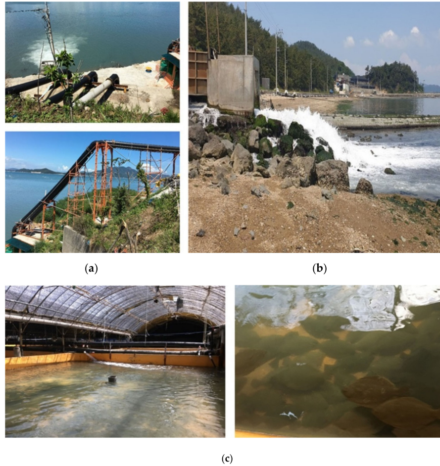
Figure 1. Fish farm facilities: (a) water supply system; (b) discharge water system; (c) fish farm.
