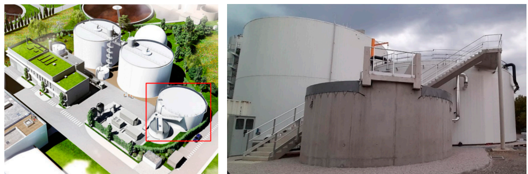
Figure 13. Three-dimensional (3D) drawing of the THP + AD sludge treatment extension project in Toulouse and photo of the IFAS ANITA Mox unit.
