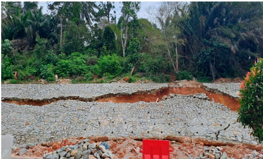
Figure S1. An image showing riprap soil slope protection in Malaysia that disintegrated or failed.
