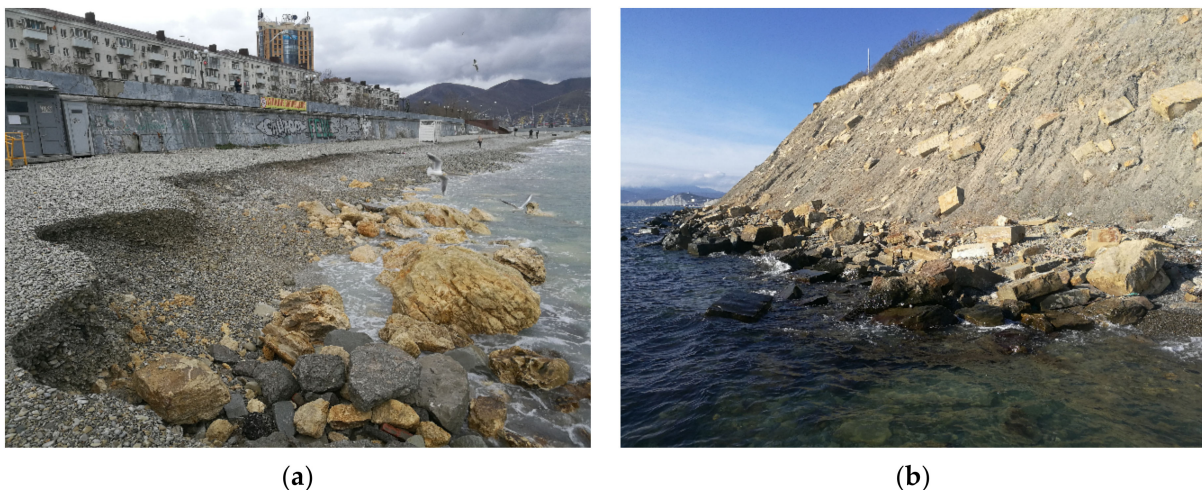
Figure 15. (a) Beach erosion in the City of Novorossiysk after a winter storm on 28 January 2021; (b) coast erosion in Shirokaya Balka near Novorossiysk due to landslide and talus processes, 4 February 2021.
