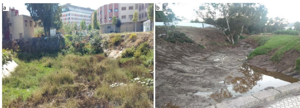
Figure 7. (a) Drainage channel not maintained or cleaned, (b) and drainage channel maintained and cleaned before the start of the rainy season (September 2021) in the city of Tangier.
