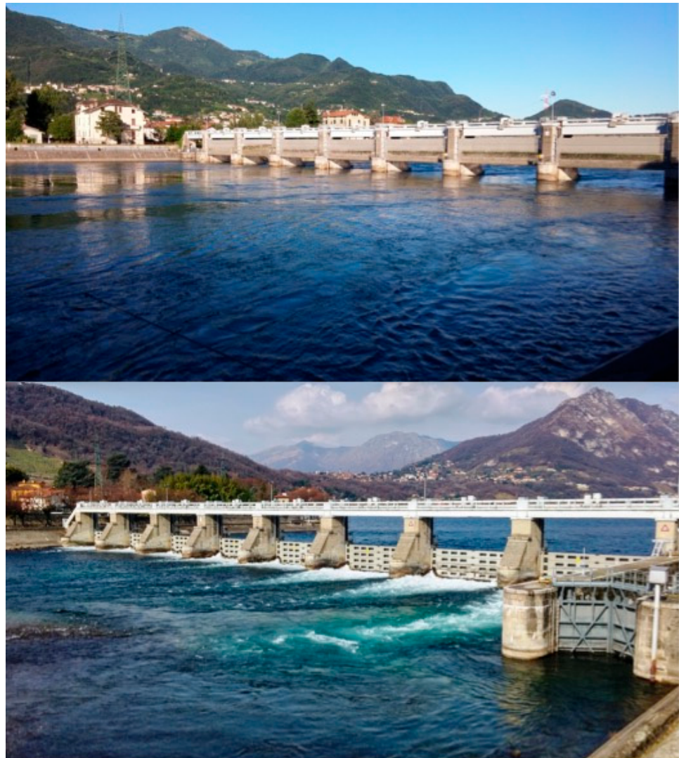
Figure 2. The Olginate dam on the Adda river at the outlet of Lake Como, seen from both sides with fully open (upper picture) and partly closed (lower picture) sluices. The navigation pond can be seen on the right of the lower picture.
