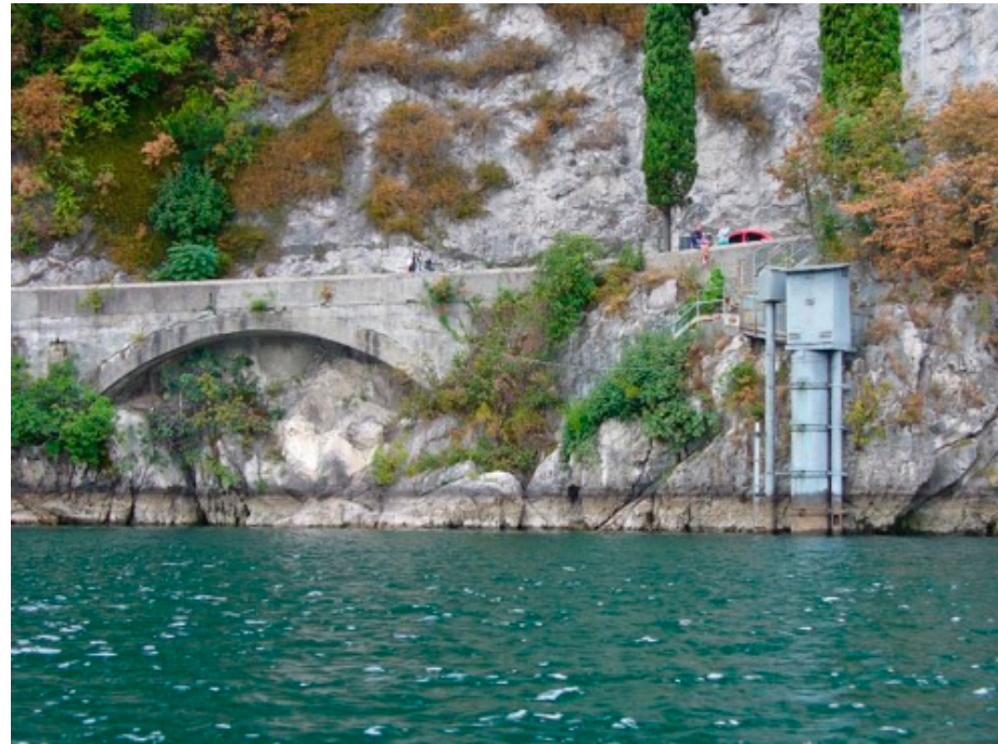
Figure 3. The hydrometric station at Malgrate 7 km upstream of the dam. A traditional floater-based water level gauge today is electronically connected to the Consorzio dell’Adda Control Centre.
