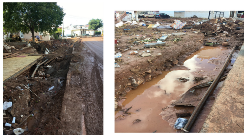
Figure 7. Example of the of the urban drainage system failure.
