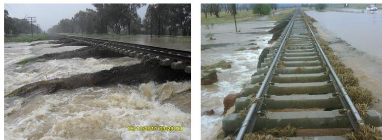
**Figure 1.** Scouring of railway ballast during flooding in the Hunter Valley, NSW, Australia, in October 2010. Copyright Australian Rail Track Corporation.
