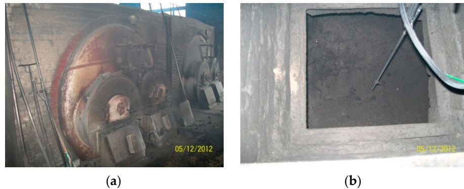
Figure 1. Steam boiler with a capacity of 2 MW in a silicate manufacturing plant in Żytkowice used for testing of the co-firing of coal with glycerine fraction; (a) view from the loading side, (b) view of the flue duct from the exhaust with a tube of gas analyzer.
