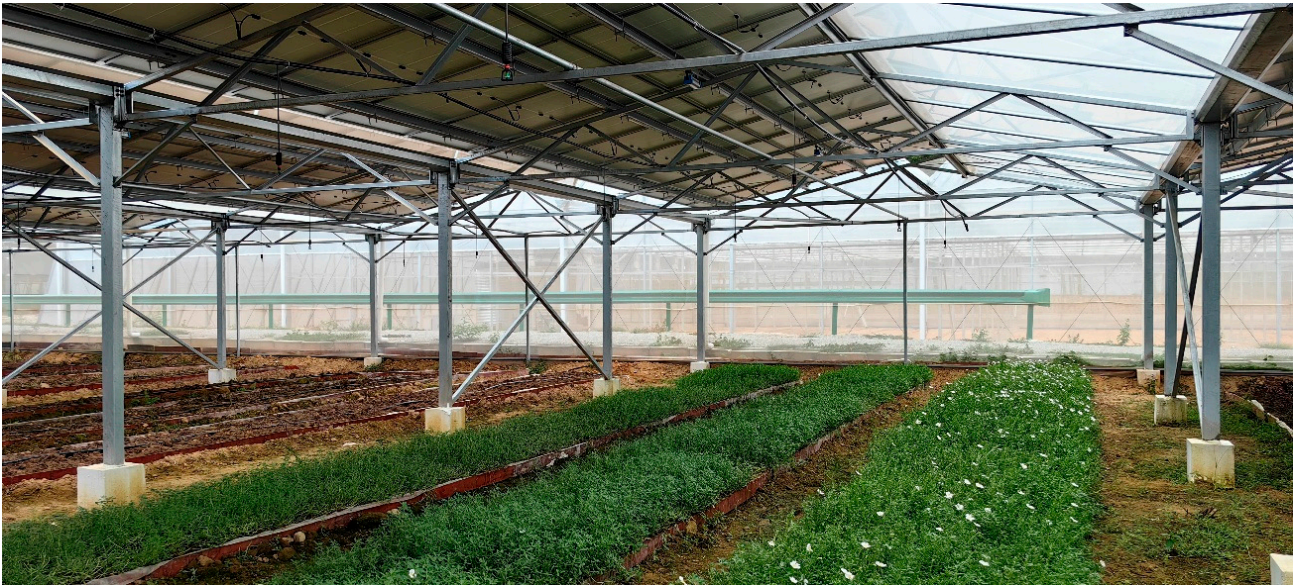
Figure 3. A real picture of the zigzag PV greenhouse.
