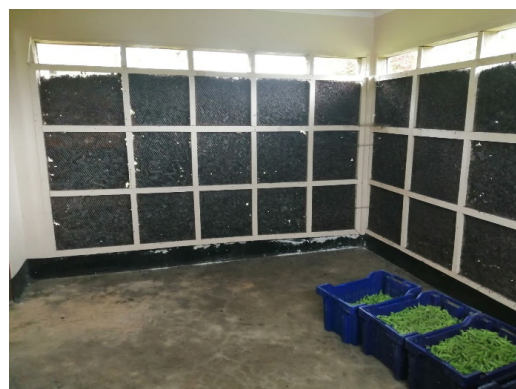
Figure 1. Charcoal Cooling Room for storage of fresh fruits and vegetables in Tanzania.
