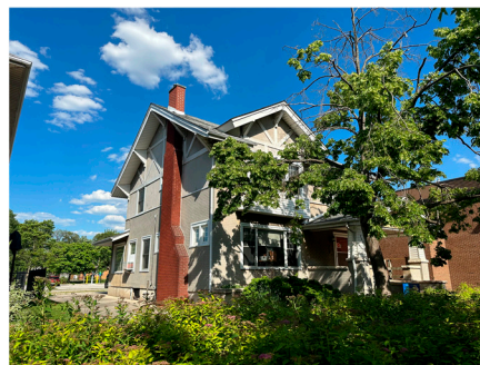
Figure 1. Detached office building assessed.
