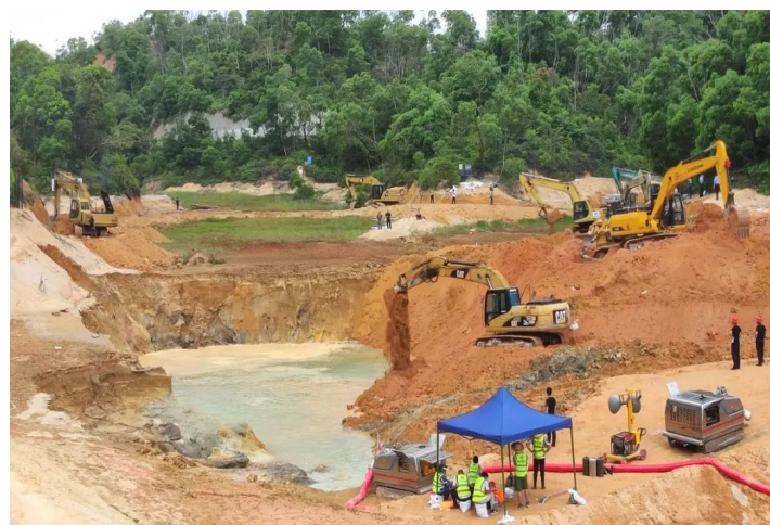
Figure 4. Rescue site cofferdam construction (Picture from: https://www.guancha.cn/politics/2021_07_17_598831_s.shtml , accessed on 18 January 2022).
