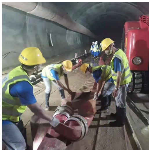
Figure 3. Rescue workers are laying out pumping equipment (Picture from: https://www.guancha.cn/politics/2021_07_17_598831_s.shtml , accessed on 18 January 2022).
