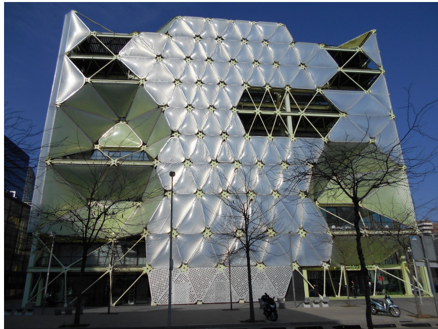
Figure 2. MediaTIC building ETFE cushions façade. Source: authors.
