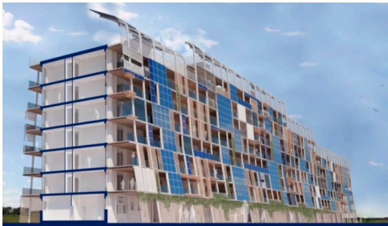
Figure 2. An example of retrofitting using the external steel frames.
