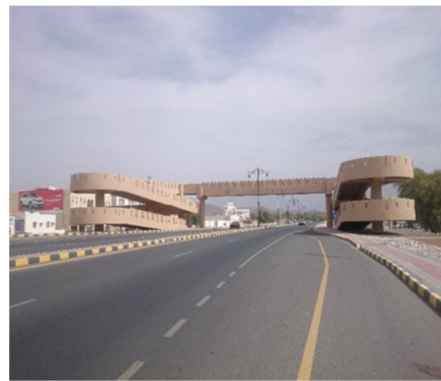
(b) A typical pedestrian crossing bridge
