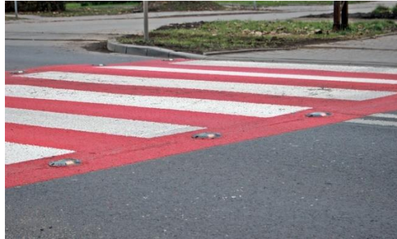
Figure 11. Advanced design of pedestrian crossings: active crossing equipped with ‘cat’s eyes’.
