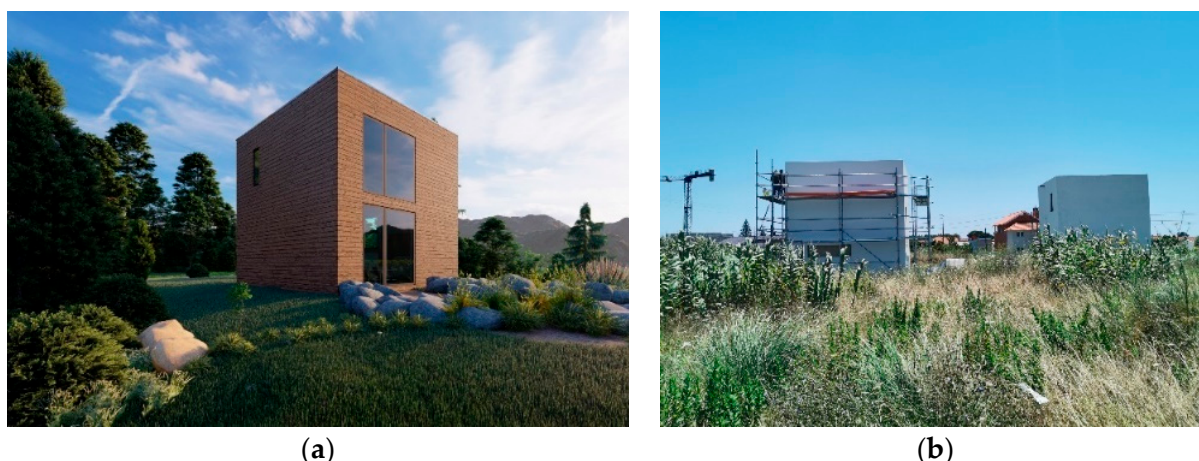
Figure 2. Tiny houses case study: (a) 3D design view of the tiny houses; (b) tiny houses under construction.
