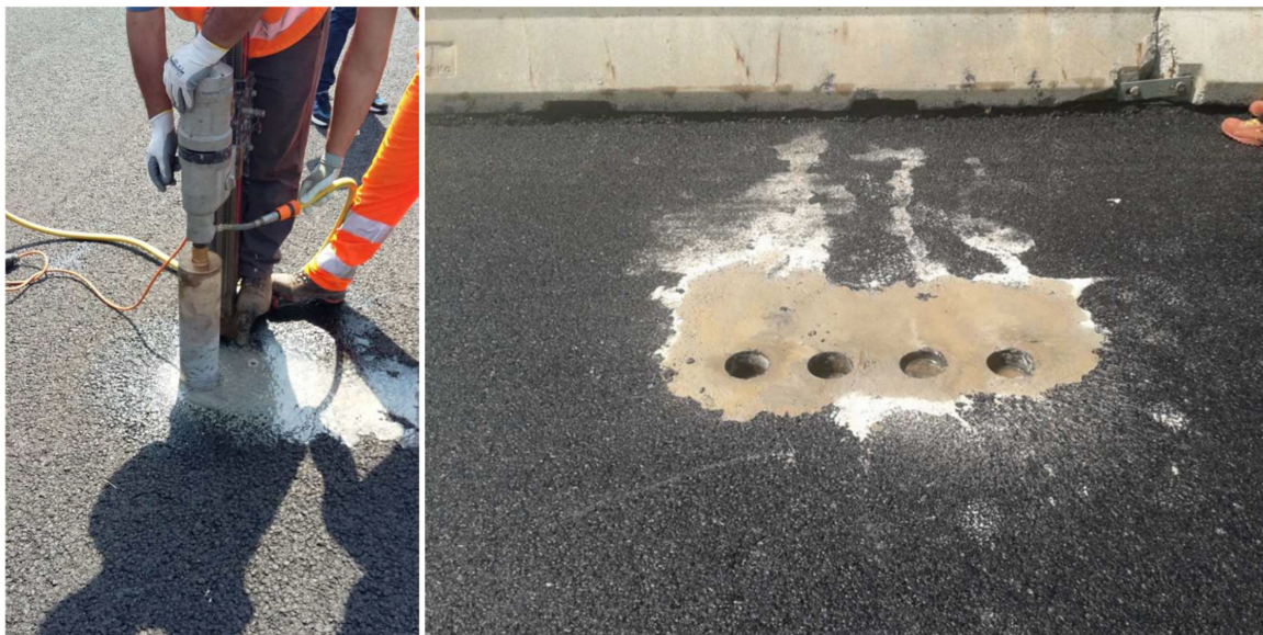
Figure 6. Taking cores for the quality assurance and in-place mixtures properties.
