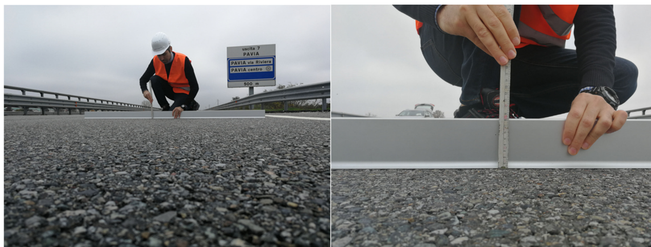
Figure 15. Rutting control of the pavement wheel paths. Autumn 2021.
