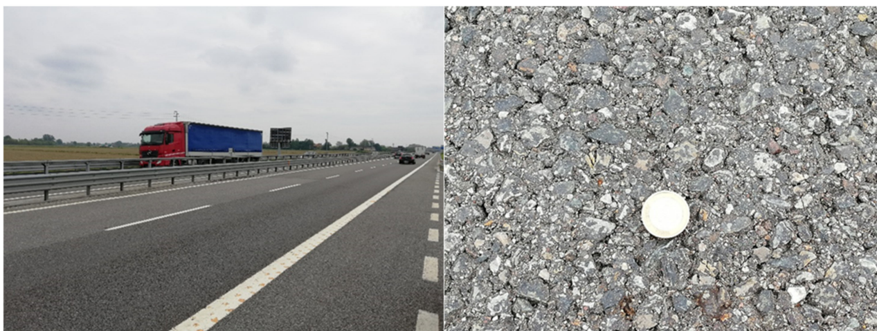
Figure 14. Pavement condition during the annual visual inspections on autumn 2021. The scale coin is EUR 1; 23.25 mm.
