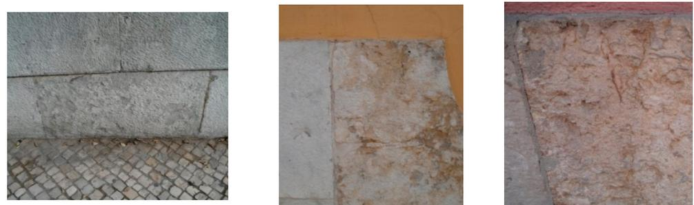
**Figure 6.** Illustrative examples of the loss of integrity anomalies observed in NSC located at the bottom wall of NSC façades.
