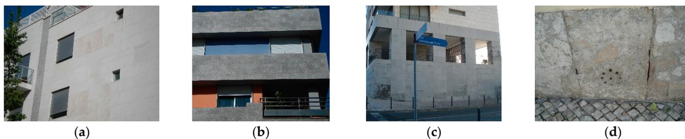
**Figure 2.** General appearance of NSC in the different degradation conditions: (a) condition A ( $S_w \leq 1\%$ ); (b) condition B ( $1 < S_w \leq 8\%$ ); (c) condition C ( $8 < S_w \leq 20\%$ ); (d) condition D ( $20 < S_w \leq 45\%$ ). No example is provided for condition E because there is no NSC in this condition in the database.
