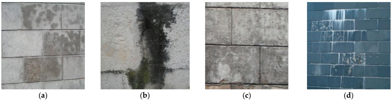
**Figure 4.** Illustrative examples of the visual anomalies observed in NSC: (a) damp stains; (b) biological colonisation; (c) dirt deposition; (d) efflorescence.
