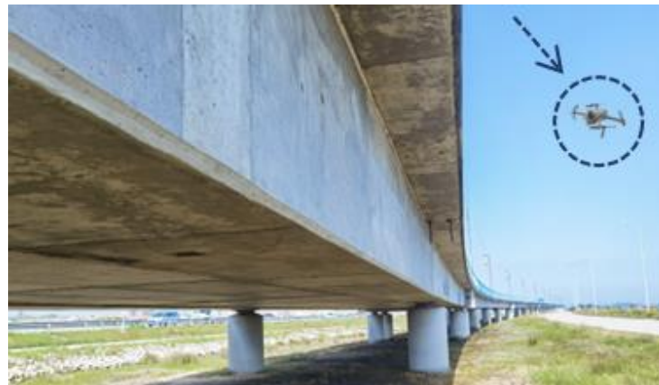
Figure 9. UAV in operation.
