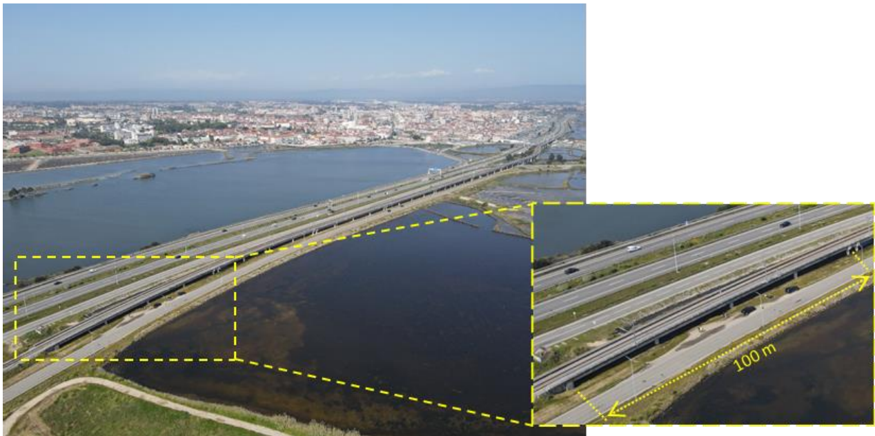
Figure 4. Extremity module of the west access viaduct of the Pirâmides bridge (Aveiro, Portugal).
