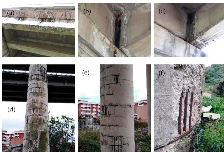
**Figure 7.** Some defects identified on PC bridges of A18 and A20 highways.
