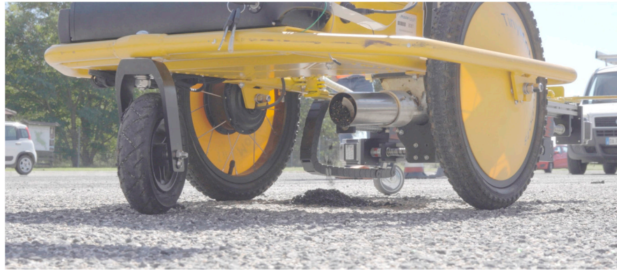
Figure 18. Pothole filling in a pothole.
