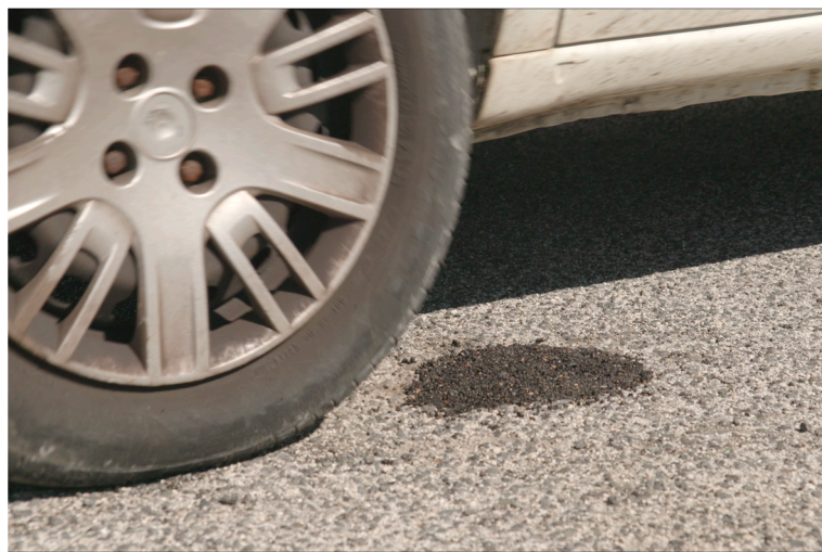
Figure 19. Mixture compaction.
