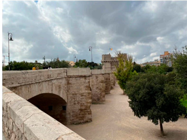
Figure 6. The Serranos Bridge in 2023 [21].
