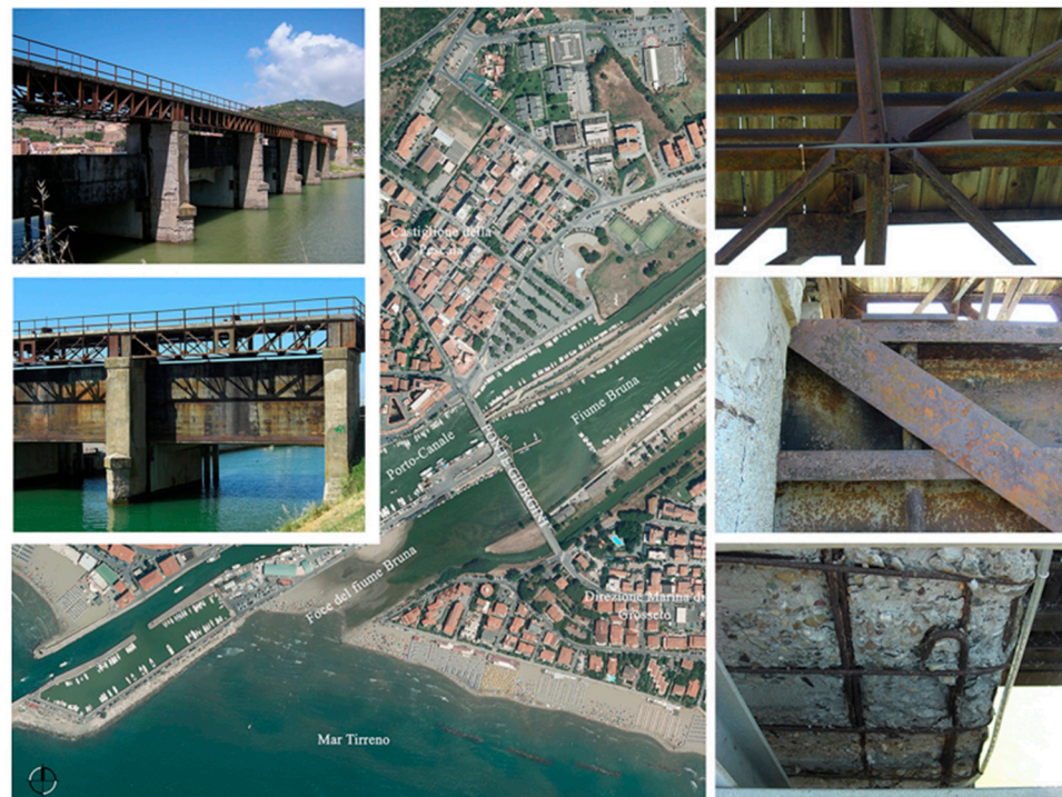
Figure 13. The Giorgini Bridge [20].
