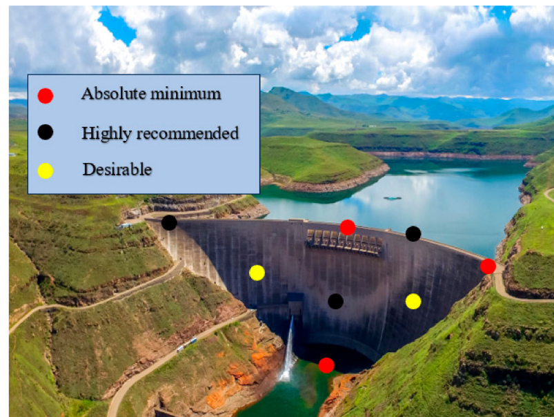
Figure 4. Proper sensor selection and installation in dams.
