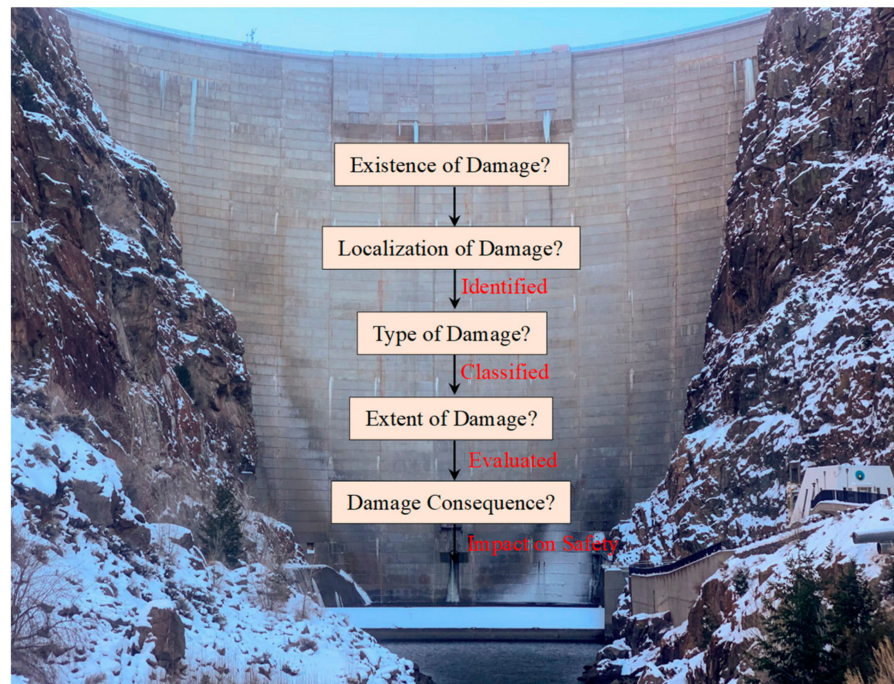
Figure 5. Damage hierarchy in dams.
