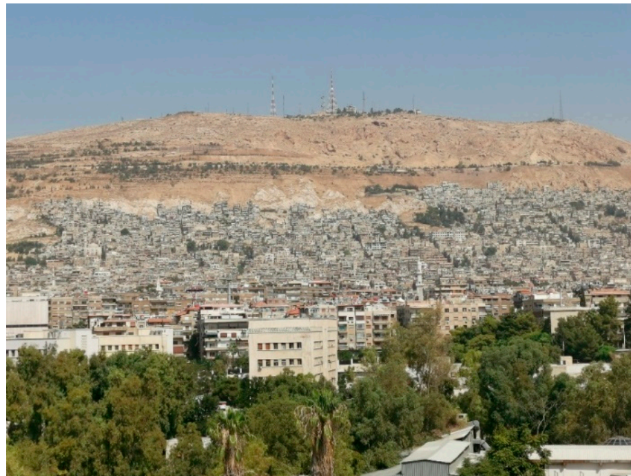
Figure 12. The expansion of slums over Mount Qasioun (September 2022).
