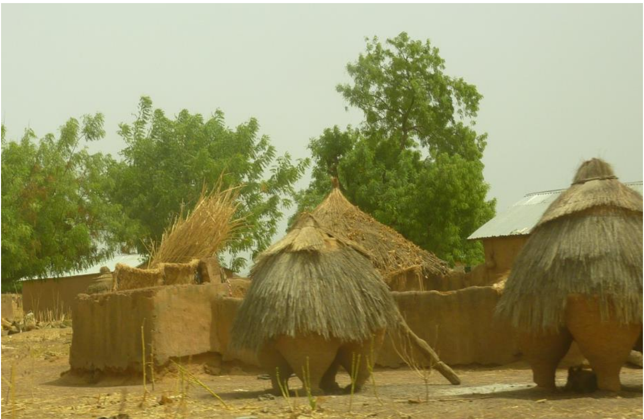
Figure 1. Architectural design and materials of traditional huts and granaries in Northern Nigeria facilitate rodent infestation (original photograph by Marianne Besson).
