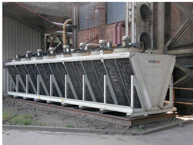
Figure 6. Fan cooling bed of furnace cooling system.
