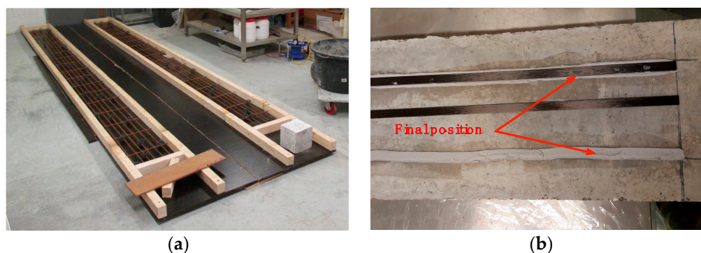
Figure 1. (a) Preparation of the specimens; and (b) CFRP bonding.
