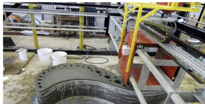
Figure 14. Large-scale 3D printing of ultra-high-performance concrete [110], reproduced with permission from Lim et al., Fabricating construction components using layered manufacturing technology ; published by Loughborough University, 2009.
