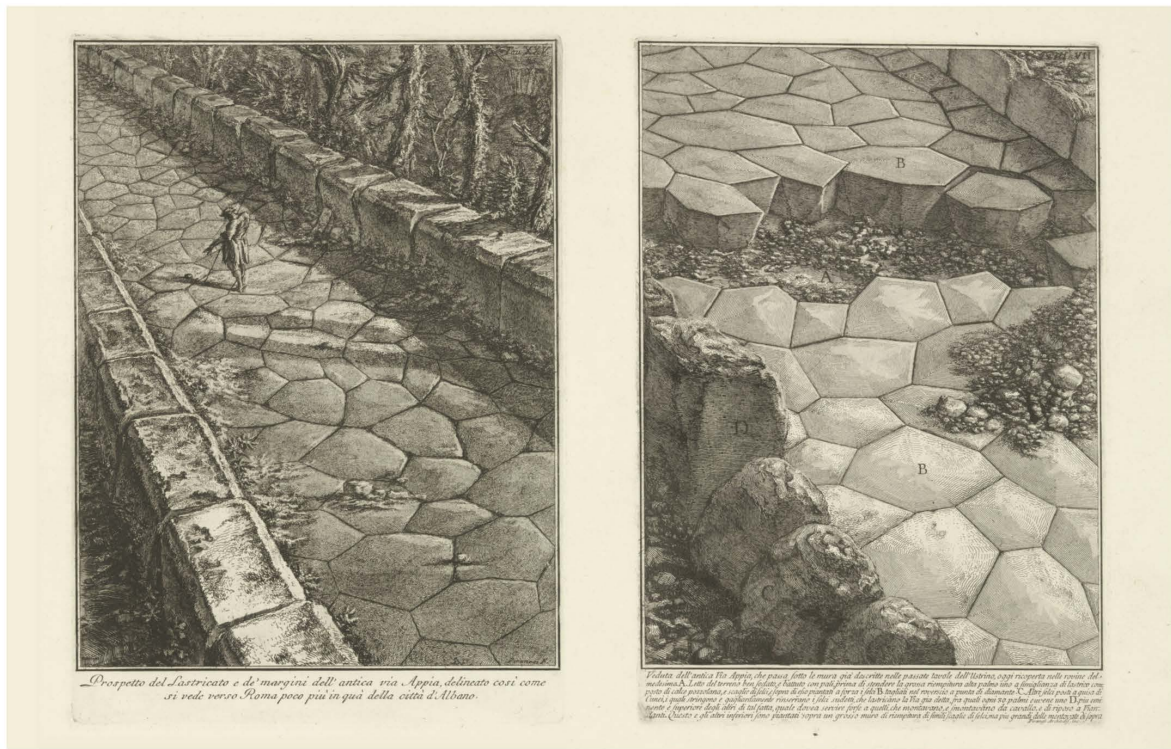
Figure 3. The Appian way: the mausoleums, and the pavement realised with polygonal blocks of mafic lava (Top). Giovanni Battista Piranesi, the pavement and the crepidines (blocks that delimit the road) of the Appian Way towards Rome shortly after the city of Albano, engraving. The Appian Way pavement is engraving on the right ( Antichità Romane , 1756—source: Europeana, https://www.europeana.eu/it , accessed on 22 November 2022) (Bottom).
