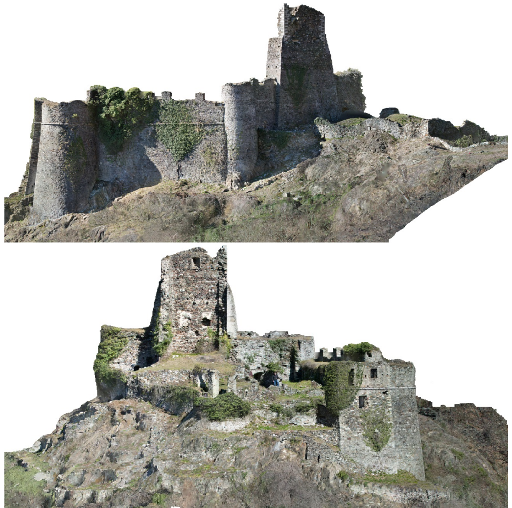
Figure 16. Two different orthophotos of the fortress elevations: South ( top ) and West ( bottom ) elevation.
