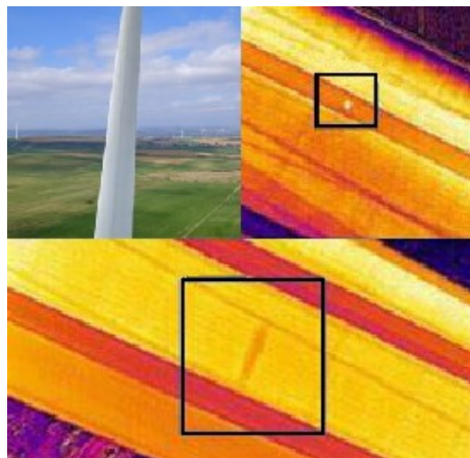
Figure 3. Internal defect of WT blade detected using infrared thermal imaging (From [42]).
