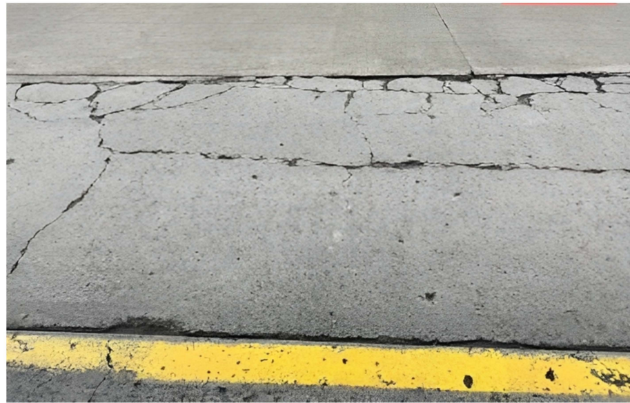
Figure 7. Pavement section captured from traditional visual inspection.
