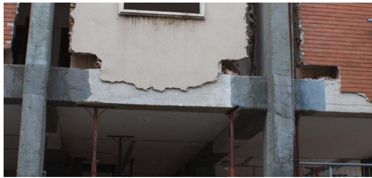
Figure 7. SRP strengthened the frame of a multistory building.
