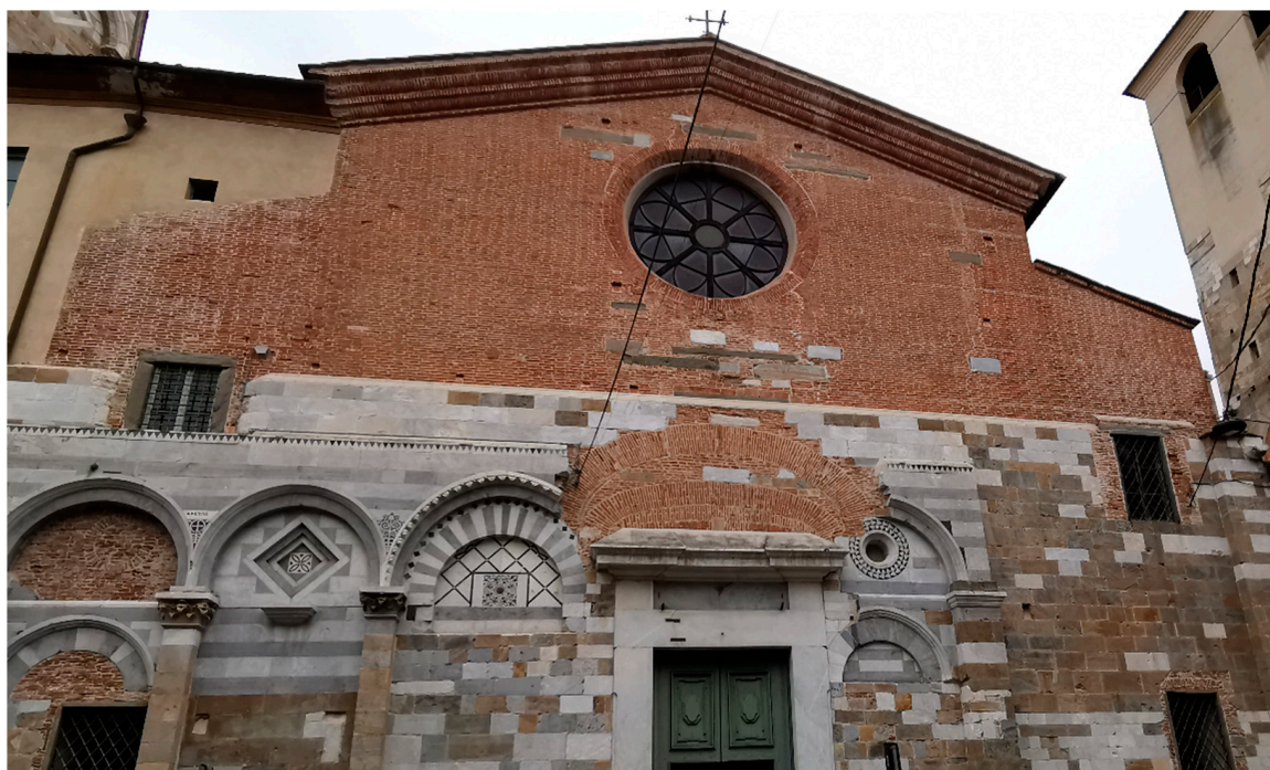
Figure 25. The actual aspect of the main façade—global view (June 2021).
