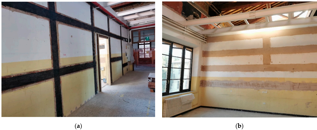
Figure 6. Composite intervention to avoid overturning of partition walls: (a) application of the composite reinforcement; (b) detail of the completed intervention.
