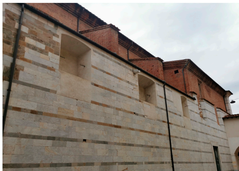
Figure 13. The south wall of St. Nicola Church.
