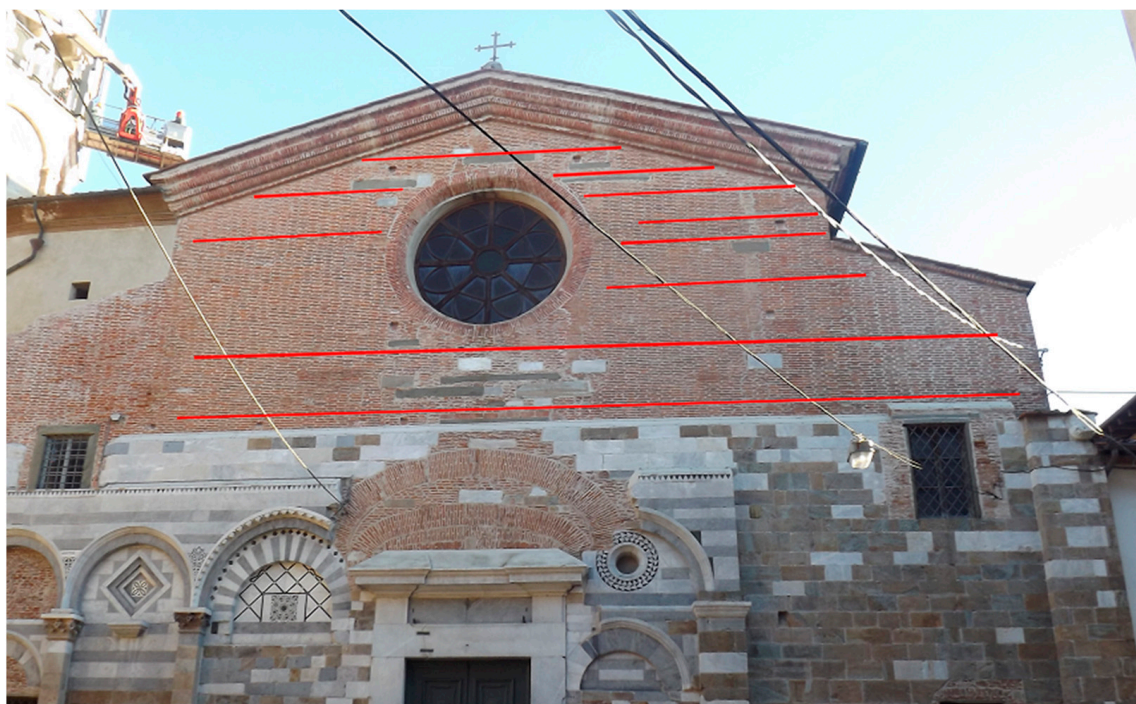
Figure 24. Strengthened brick courses of the main façade.
