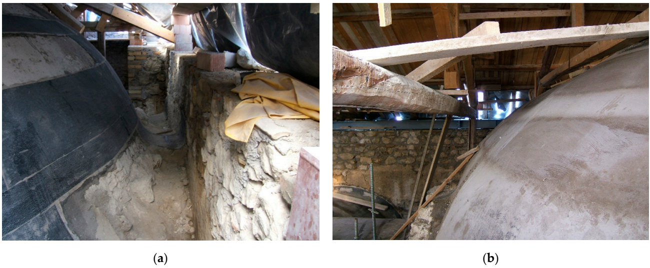
Figure 4. Composite strengthening of a dome vault: (a) detail of the composite reinforcement; (b) detail of the completed intervention.
