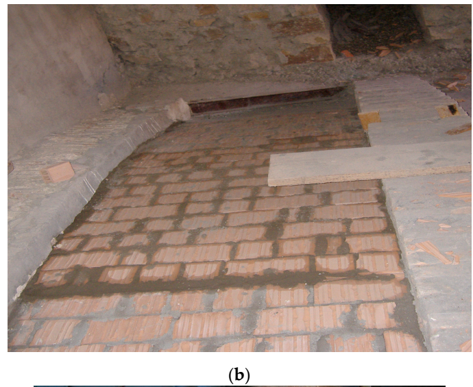
Figure 4. Composite strengthening of a dome vault: (a) detail of the composite reinforcement; (b) detail of the completed intervention.
