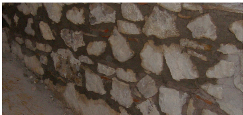
Figure 8. Application of the indentation technique: strengthening of uncoursed rubble masonry wall.
