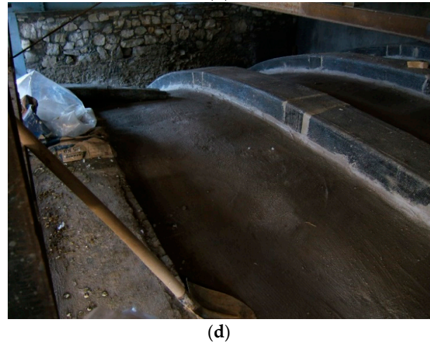
Figure 5. Composite strengthening of a partly collapsed ribbed barrel vault: (a) detail of the collapsed part; (b) reconstruction of the collapsed part; (c) detail of composite reinforcement; (d) detail of the completed intervention.
