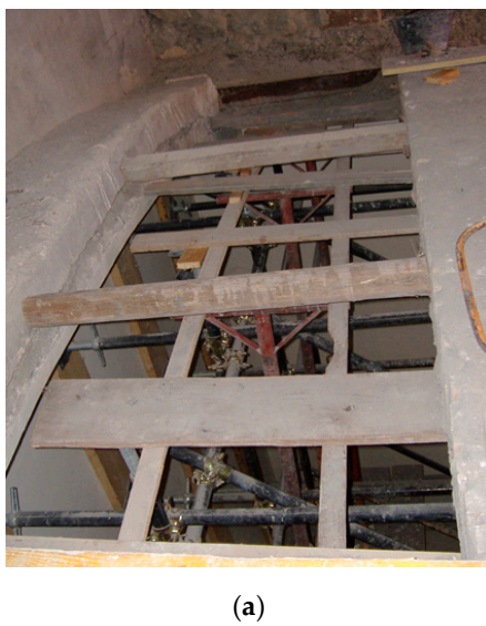
Figure 4. Composite strengthening of a dome vault: (a) detail of the composite reinforcement; (b) detail of the completed intervention.
