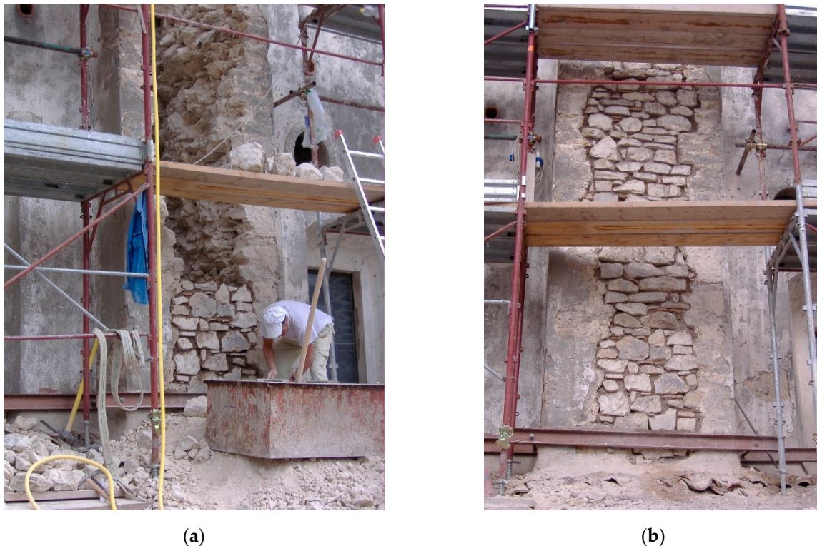
Figure 7. Application of the indentation technique to the strengthening of a parastas: (a) during the intervention; (b) at the end of the intervention.
