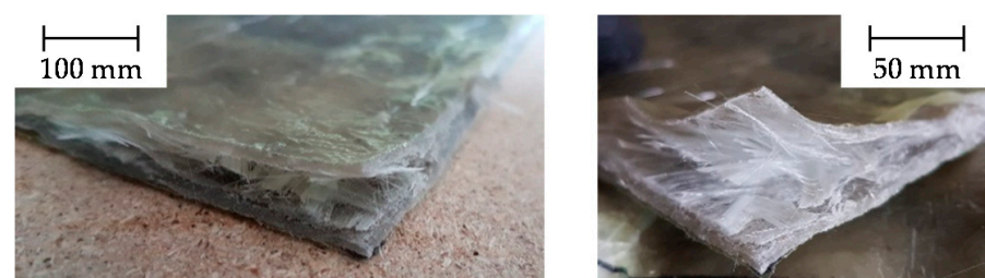
Figure 1. Inadequate fiber impregnation at the edges of the preform.
