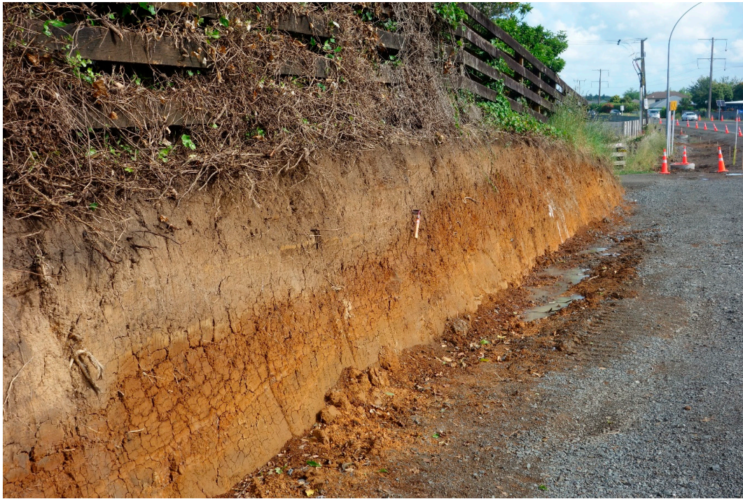
Figure 2. Exposure of Kainui silt loam on Gordonton Road practically opposite the intersection with Thomas Road ( 37^{\circ}43'55'' S, 175^{\circ}17'15'' E), northern Hamilton (Figure 1). The two-storeyed nature of the Kainui soil is striking, with the pale composite coverbed of late Quaternary tephra contrasting with the paleo-surface of the underlying dark reddish-brown clay-rich Hamilton Ash beds. The profile looks a lot like the ‘strong texture-contrast’ or ‘duplex’ soils that are common in Australia, e.g., [40,41] and elsewhere but it has quite different origins. The wavy to irregular boundary (marked by the small cutting tool c. 30 cm long) likely reflects tree-overturn hollows and mounds [42] (cf. [43]) (Figure 3). The thickness of the coverbed here—each part of which has been an ‘A’ horizon at the land surface at some time since c. 50 ka—ranges from a maximum of c. 0.7 m (foreground) to c. 0.3 m. Photo: D.J. Lowe.
