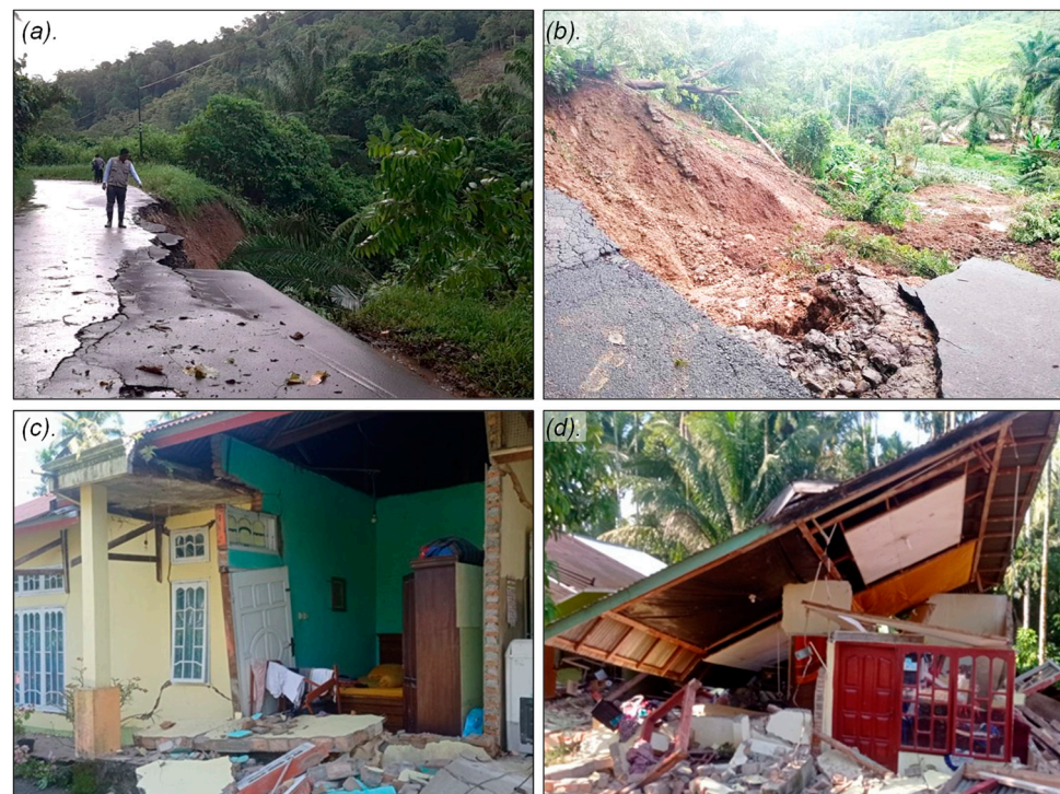
Figure 2. Damage of the Pasaman earthquake: (a) landslide, (b) road damage, and (c,d) building structural damage.
