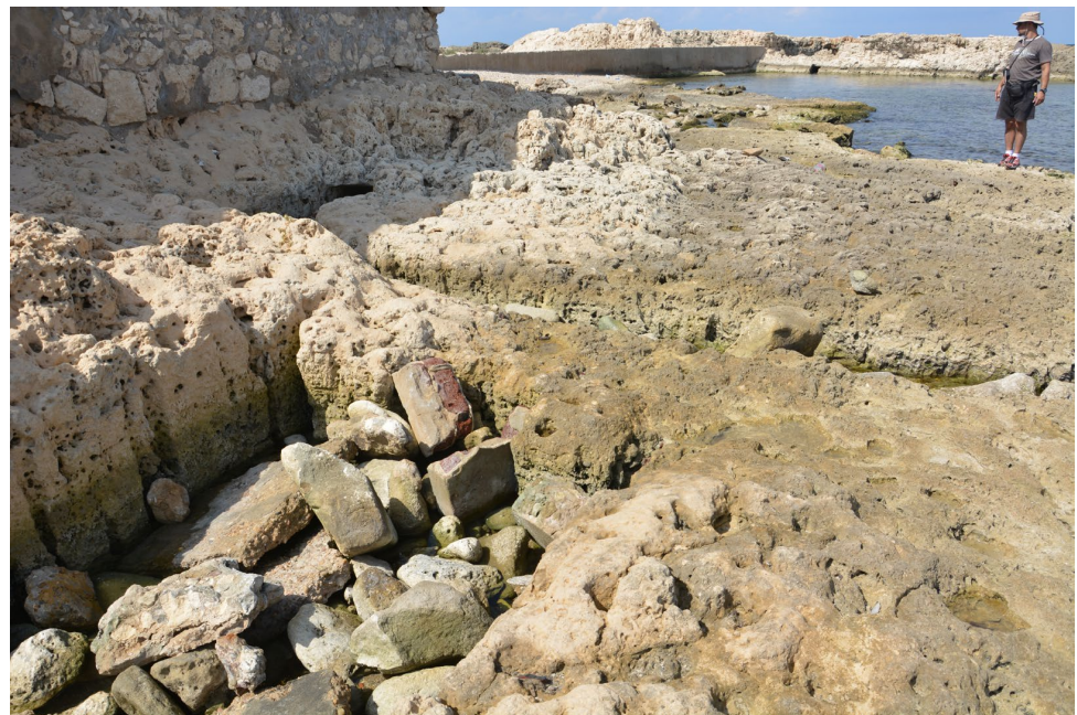
Figure 2. Channel that enabled the transportation of fresh water into the Montazah fish tank of Alexandria, Egypt.
