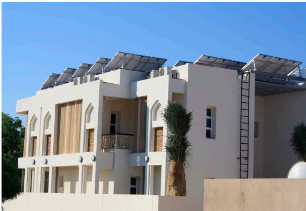
Figure 14. SQU Eco-House equipped with a 20kW PV Array which can supply both to Grid and to the household electrical commodities. The RES here works as distributed energy resource (DER) for the SG.
