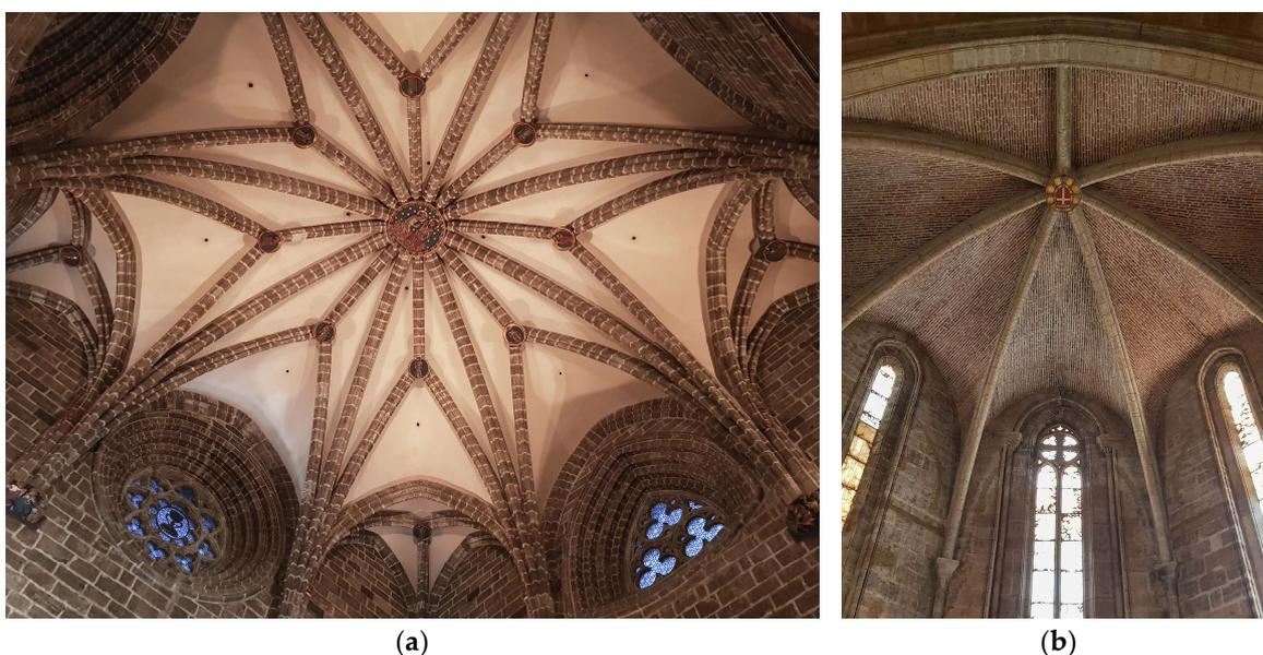
**Figure 3.** (a) A view of the star-shaped ribbed vault of the Chapel of the Holy Chalice in Valencia Cathedral (source: Renan Rolim (2019)); (b) a view of the ribbed vaults of the presbytery of the church of San Juan del Hospital (source: Renan Rolim (2023)).
