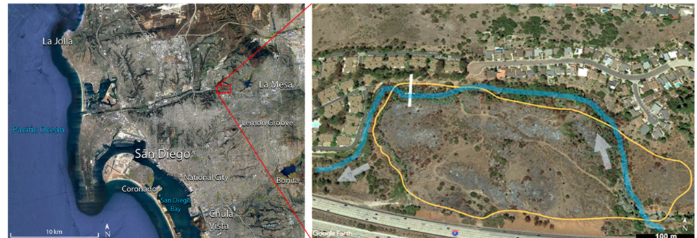
Figure 1. The study area, Alvarado Creek, is located in San Diego, California ( left image ). A Google Earth Image of the study reach (in blue) in Alvarado Creek ( right image ). The arrows indicate the direction of streamflow. The orange line denotes the Del Cerro fire perimeter. The solid white line is the approximate location of a transect established in the study site where soil samples were collected. The pebble count method to estimate stream-bed material was conducted approximately along the dotted line, where the transect intersects the study reach.
