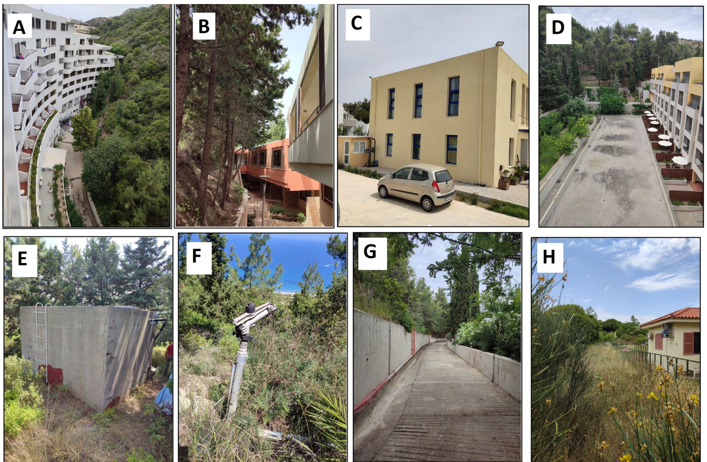
Figure 7. (A) Excessive Forest fuel consisting of pines ( Pinus brutia ) and shrubs, which are in contact with a building greatly increase the WREIS sub-indices 1 and 3. (B) Increasing of WREIS sub-indices 1 and 3 due to the presence of trees and dry branches that abut building balconies. (C) The building balcony door is not protected by a shutter and its glazing is single, greatly increasing WREIS sub-index 2. Sub-index 2 is significantly reduced due to the absence of flammable materials on the building exterior and its roof. (D) WREIS sub-index 3 is reduced due to the large distance (15 m) of the building's external perimeter from the neighboring forested area. (E,F) Independent water tank with its own pump and backup power source connected to water cannons can reduce the WREIS sub-index 4. However, the presence of dense forest vegetation consisting of pines, shrubs, and dry vegetation over 20 cm in height, significantly increases the values of WREIS sub-index 3. (G) The construction of a road to provide access for firefighting vehicles around this tourist facility, as well as the establishment of a permanent fire suppression system consisting of an autonomous water tank with a capacity of 100,000 L, reduces WREIS sub-index 3 due to the interruption of forest fuel continuity, as well as the WREIS sub-index 4 (Fire Protection Systems) and sub-index 5 (Community Infrastructure). (H) WREIS sub-index 2 is significantly reduced due to the absence of flammable materials on the building exterior and the roof of the building. However, the presence of dense grass and shrub vegetation significantly increases the values of the WREIS sub-index 3.
