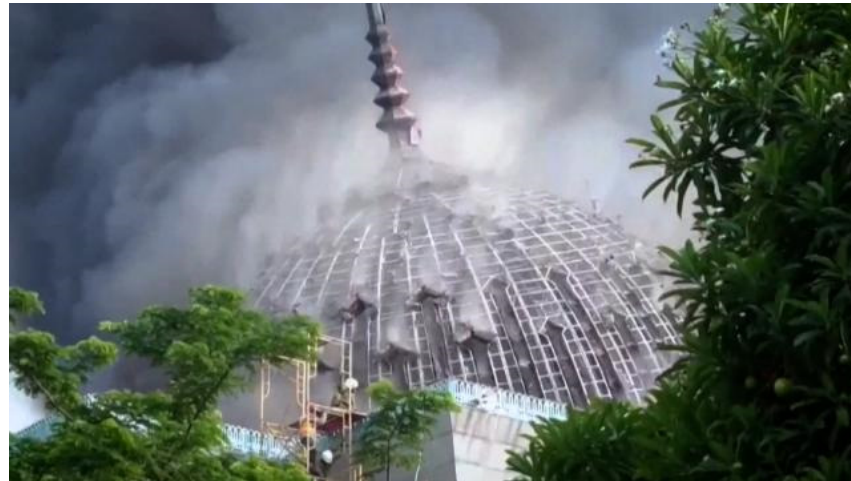
Figure 3. Collapse of a dome in Jakarta due to fire [5].
