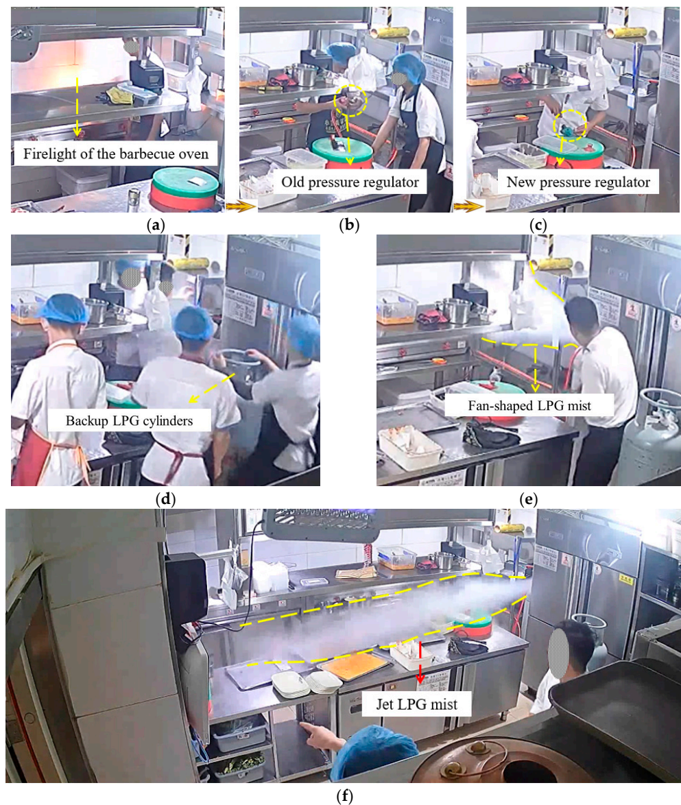
Figure 7. LPG leakage process caused by human operation error: (a) turning on the barbecue oven; (b) removing the old pressure regulator; (c) installing the new pressure regulator; (d) first small-scale LPG leakage; (e) second LPG leakage; (f) large-scale LPG leakage.
