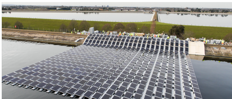
Figure 5. Array deployment using a ramp. Reprinted with permission from [14]. 2019, World Bank.
