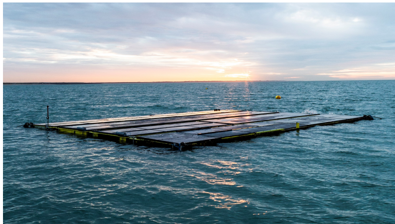
Figure 9. Marine FPV installation in the Dutch North Sea ( 56^{\circ} N, 3^{\circ} E). Reprinted with permission from [75].
