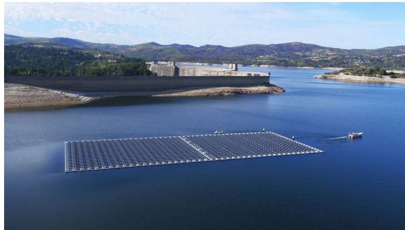
Figure 7. First HPP FPV hybrid system installed on Alto Rabagao reservoir, Portugal in 2017 (41.7° N, 7.9° W). Reprinted with permission from [14]. 2019, World Bank.
