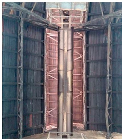
**Figure 10.** Roof construction of the Roundhouse Railway Workshop.
