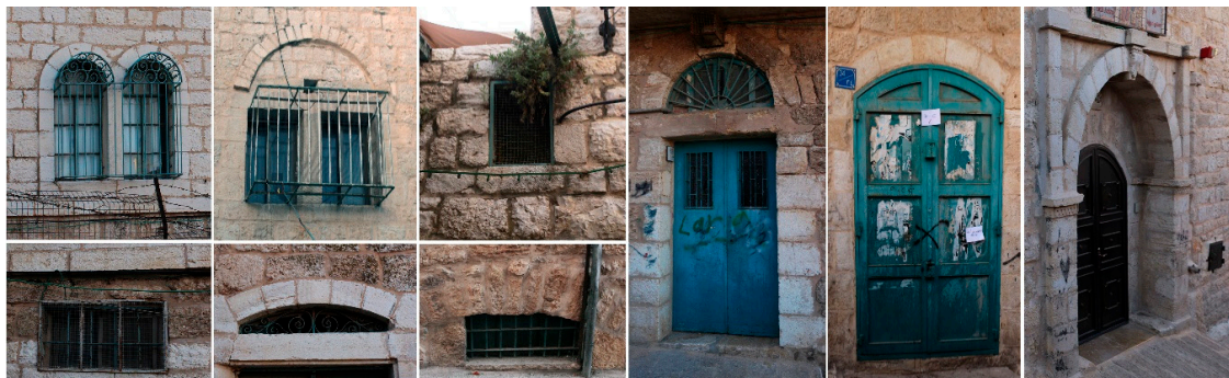
Figure 10. Constructive elements and opening solutions, original or from subsequent interventions.
